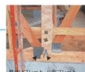
Brace end & Column base metal joint retrofitting
