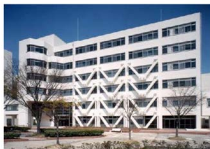
Seismic Retrofitting (Toyohashi University of Technology)
