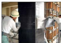
Retrofitting by carbon fiber sheet
