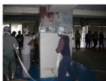
Retrofitting by polyester fibersheet
