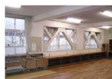
Retrofitted by V shaped steel brace
