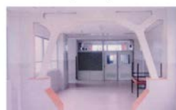
Retrofitted by Mansard shaped steel brace
