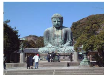
Kamakura statue was rehabilitated in 1960 adopting sliding foundation.
