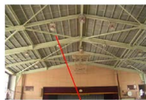
Horizontal brace Retrofitting of roof surface by horizontal bracing
