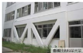
Retrofitted by brace
